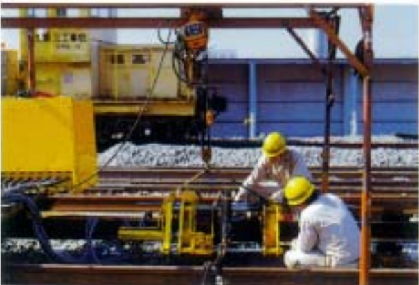
On Track Welding Method
